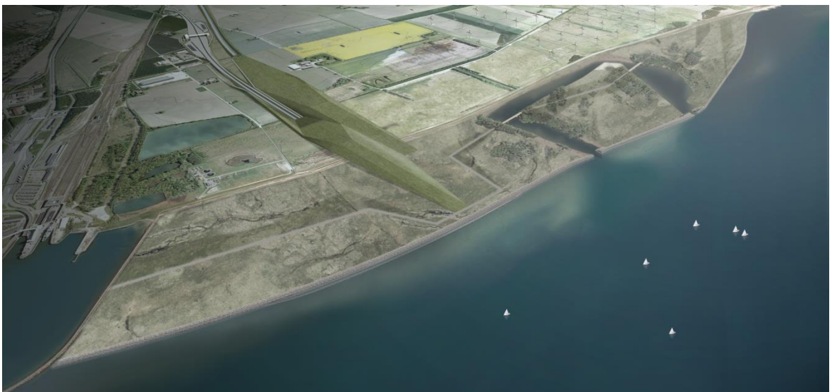
Figure 6.12 Portal buildings and ramps on the Lolland side.
