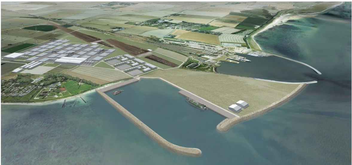
Figure 6.15 Fehmarn construction site.
