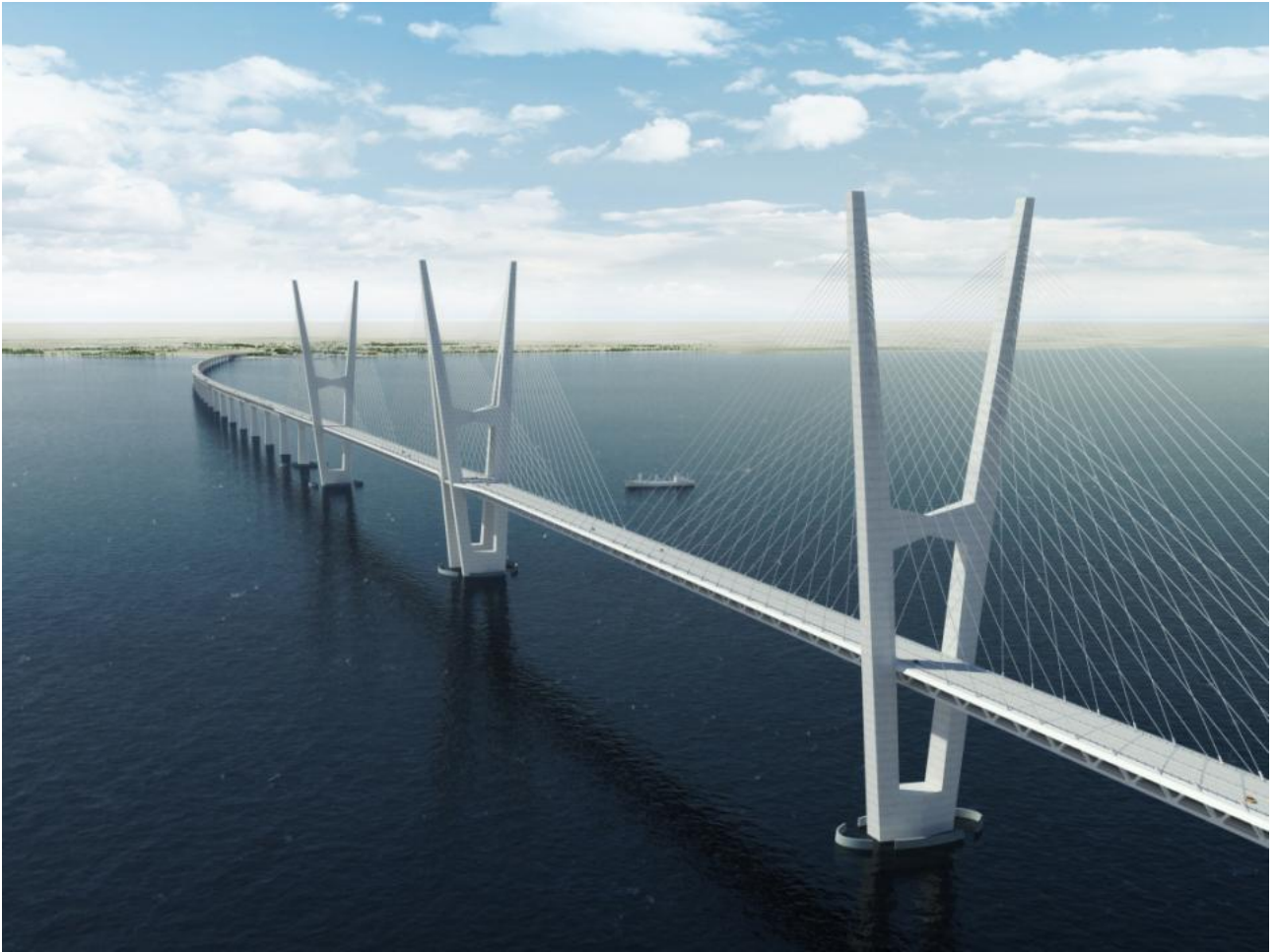
Figure 6.8 Cable Stayed Bridge.
