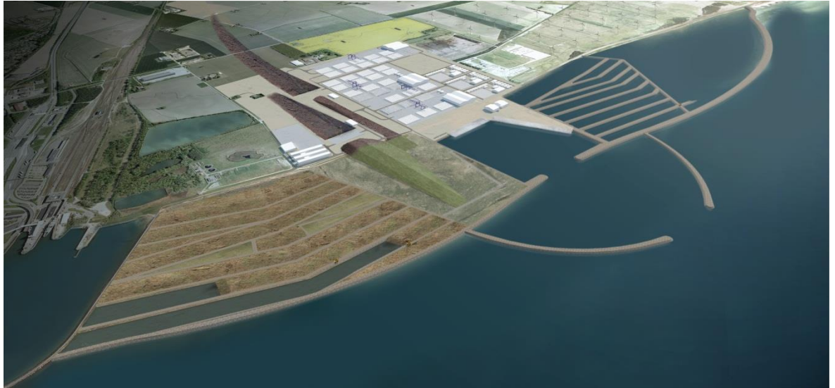
Figure 6.16 Lolland construction site.
