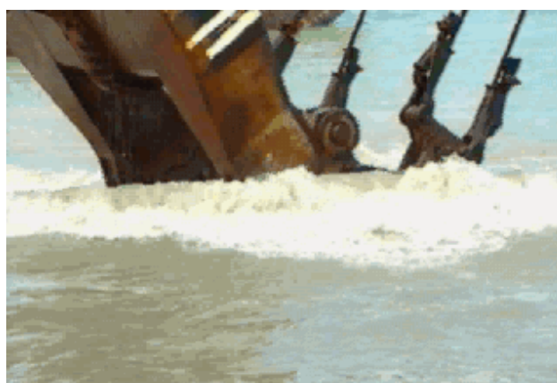
Example of dredging operation
