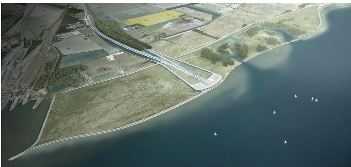
Figure 2.5 Tunnel portal area at Lolland
