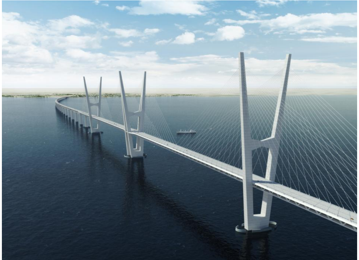
Figure 2.8 Main bridge part of the cable stayed bridge
