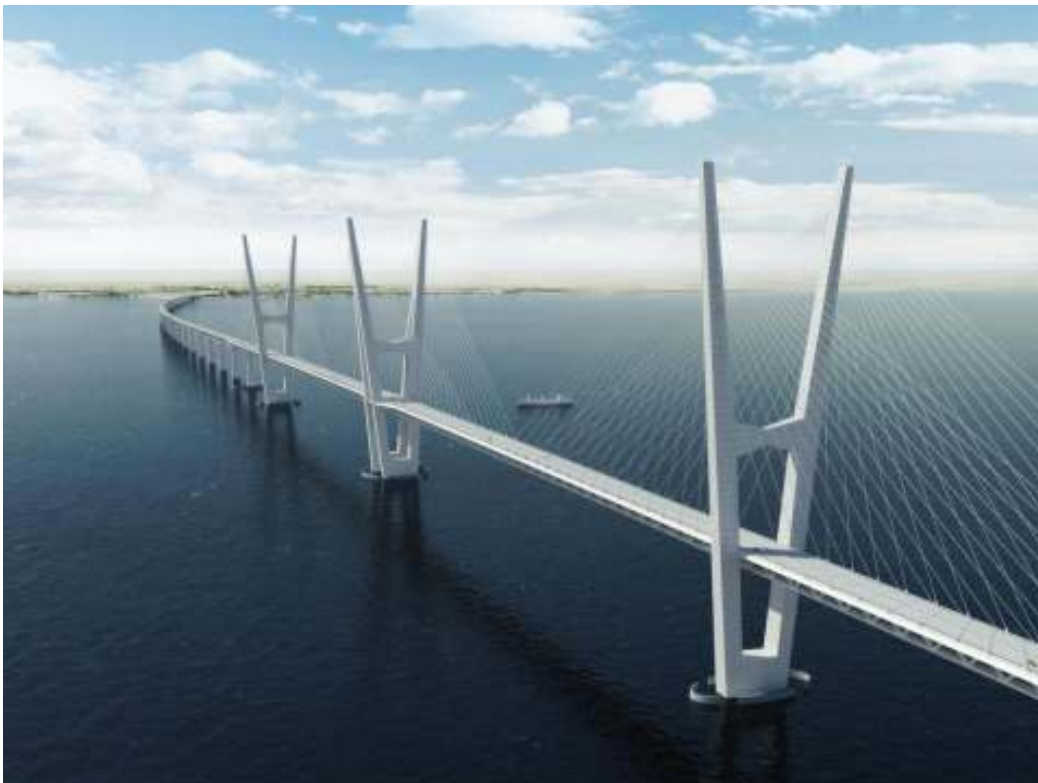
Figure 10.1 Cable stayed bridge.
