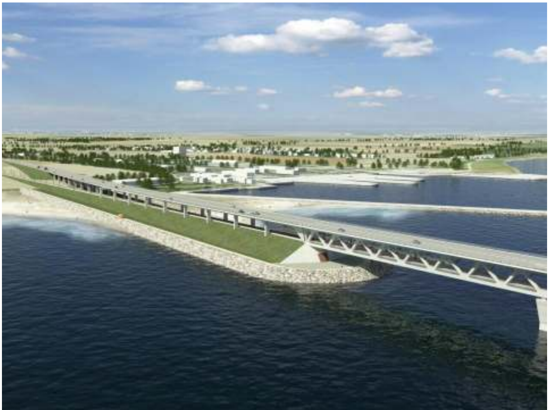
Figure 10.2 Peninsula of a cable stayed bridge at Lolland.
